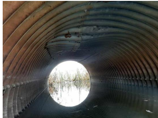
Fig 1: Damage to Culvert
